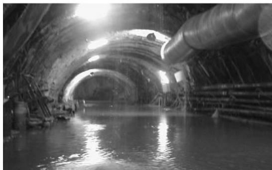
Fig.17 The Vast Amount of Groundwater in front of the Excavation Face
